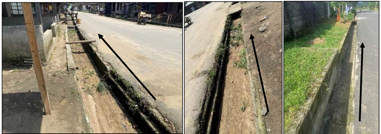
Fig. 4.3. Municipal drainage systems in Okochiri. Municipal sewage was not observed in the community's drainages. The arrow shows the flow direction.
