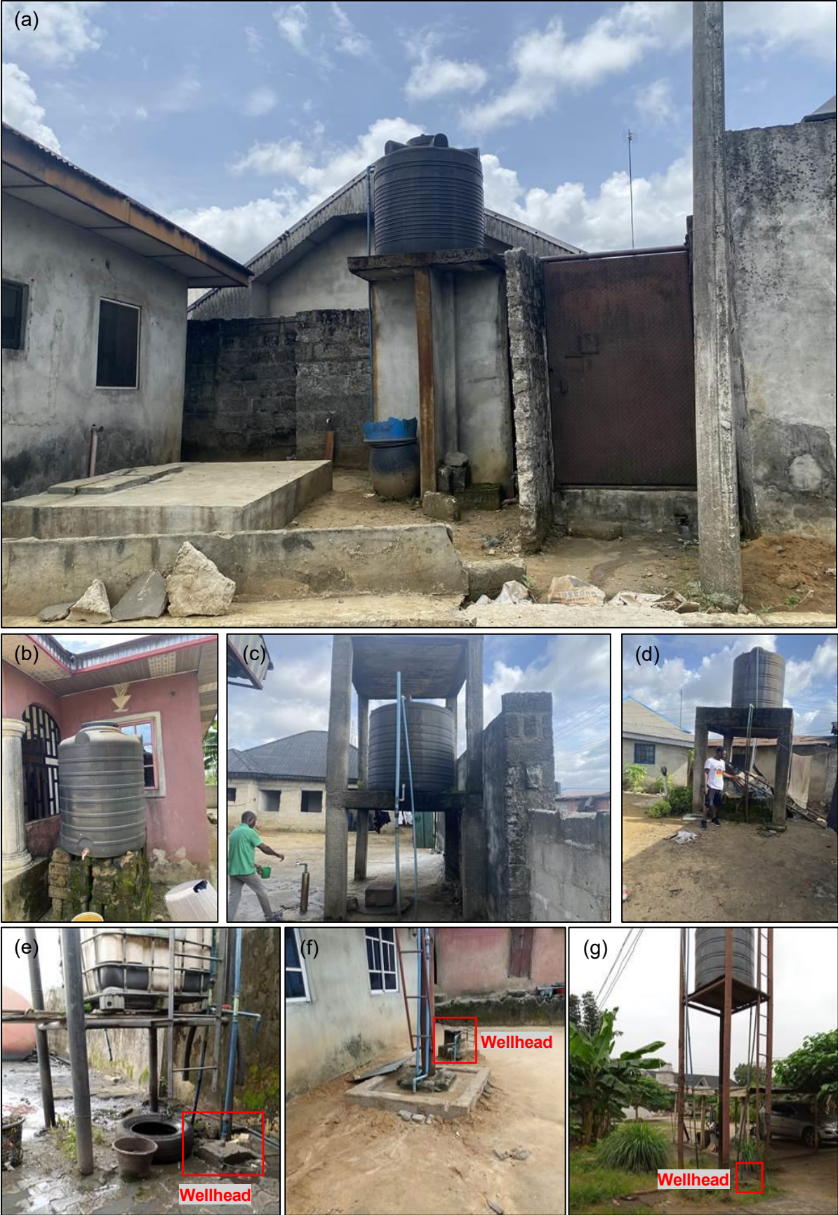
Fig. 4.4. The overhead storage tank for drinking water in the (A) Alode, (B), (E), and (F) Okochiri, (C), (D), and (G) Ogale.
